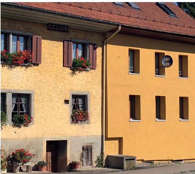
The facade of the building on the right has been newly insulated, but in the process the history of the house has been lost.
