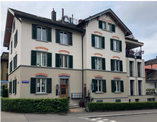
10-year-old Aerogel facade given no maintenance
