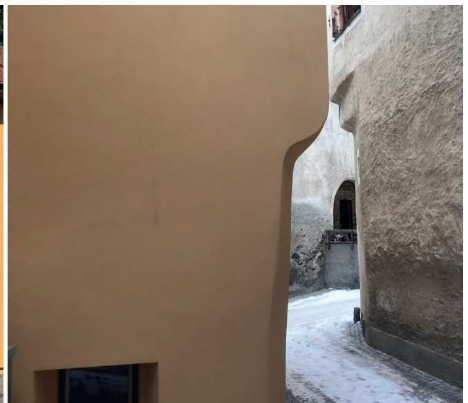
Here the facade created with Aerogel insulating render is telling a story that is still understandable in its context.
